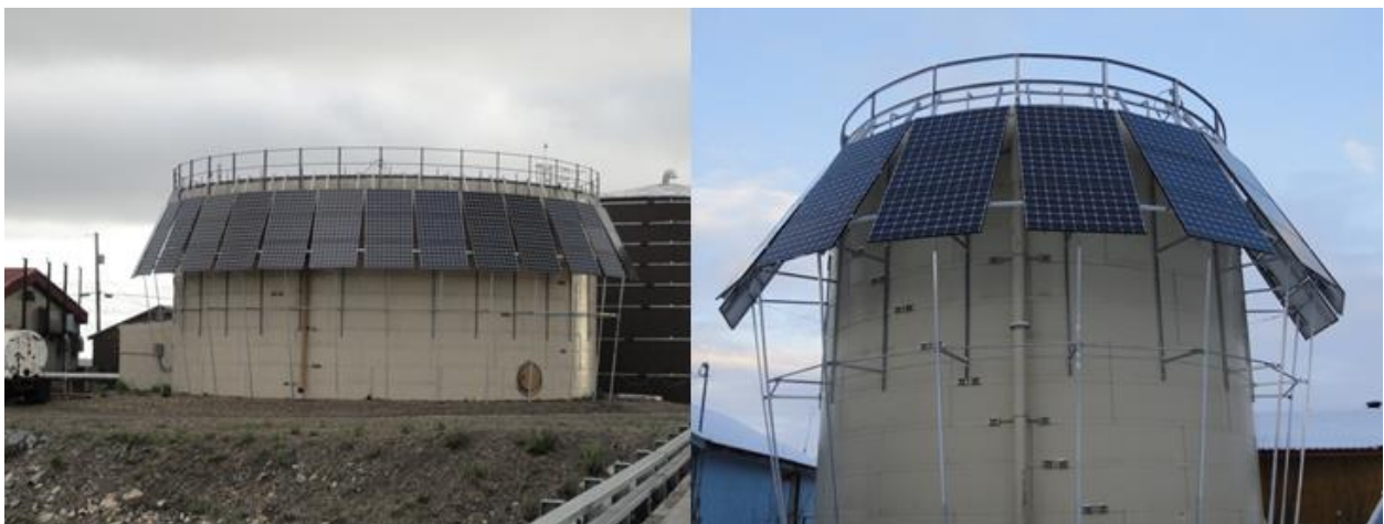
Figure 2. Circular Arrays on Deering (L) and Kobuk (R) Water Towers (credit: R. Bensin)
